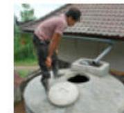
**precast ferrocement septic tank**
